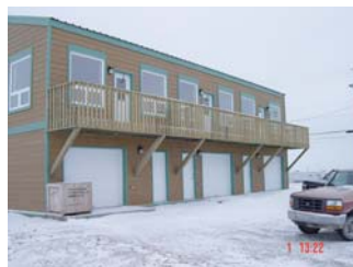
A high-end triplex recently constructed in Cambridge Bay for healthcare workers
