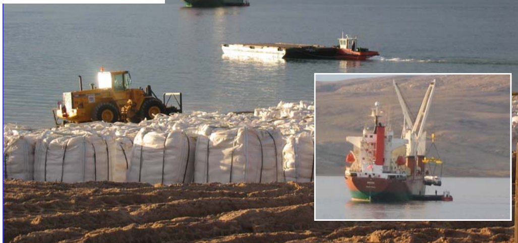
Nuna Logistics mobilizing at Milne Inlet (Baffinland Iron Mines Corporation)
